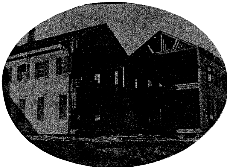
Moving day for Hough Street School in 1905. The frame building was cut into four sections and moved. Two sections became homes on Dundee Avenue, and one later became The Greenery Restaurant on North Avenue.
