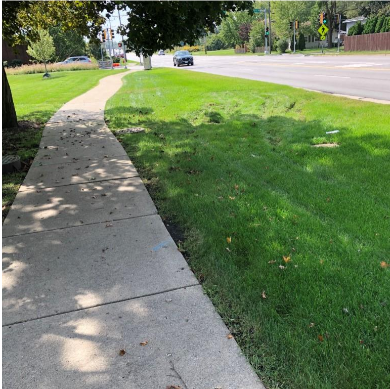
Figure 8: Area of Flooding at North Sidewalk
