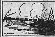
Cars Filling Embankment from Cableway.
